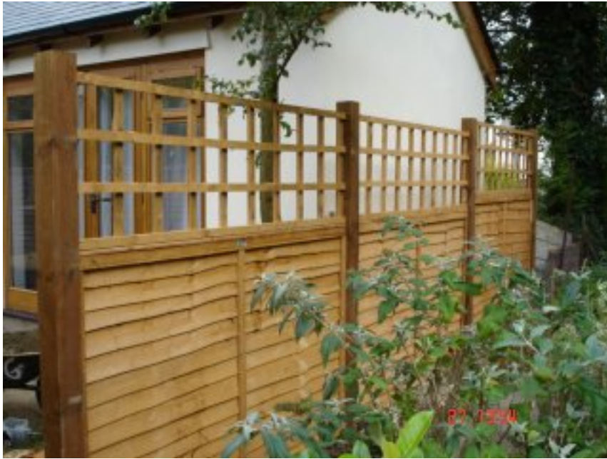
Panel fence finished with trellis.
