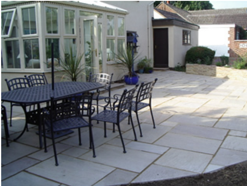
New paved area including retaining wall for raised flower beds.
